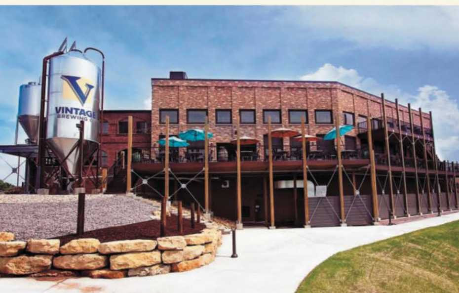
Click here for more photos and a time lapse video of the project from the ground up.
